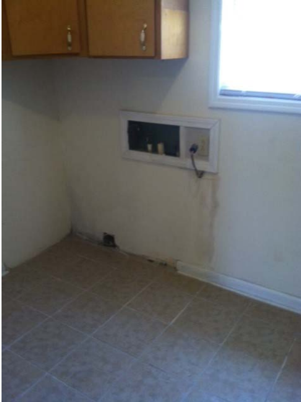
Laundry/Utility Room Renovated
