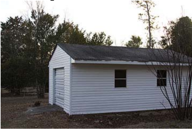
Side of Garage Renovated
