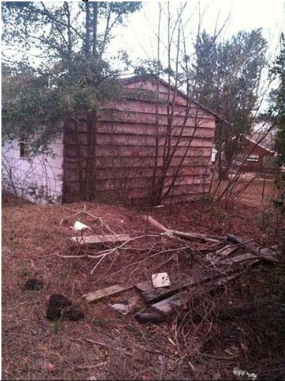
Back of Garage
