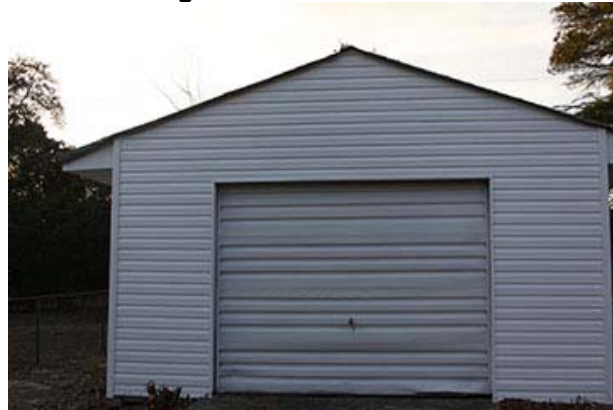
Front of Garage Renovated
