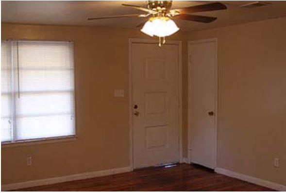
Front Room Renovated
