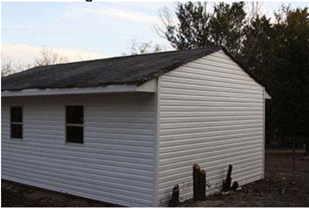
Back of Garage Renovation
