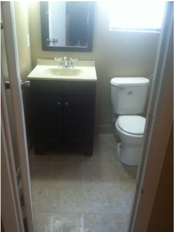
Master Bathroom Renovated
